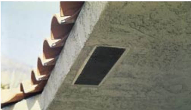
Vents located near the roofline rather than the wall.
