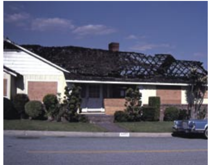
The burned roof demonstrates that nonflammable roofs are a key to fire safety.
