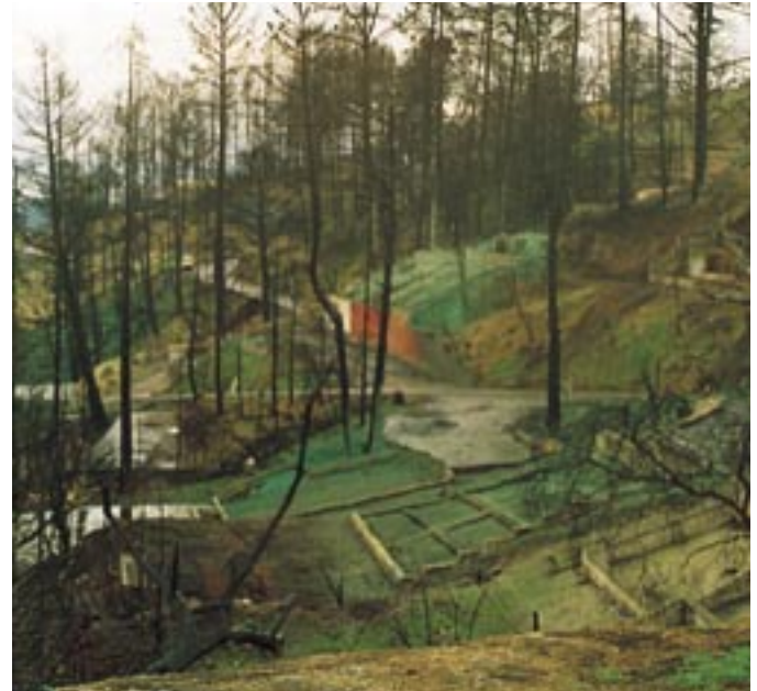
Post-fire emergency control measures are effectively used to protect the foundations/building sites of burned homes.
