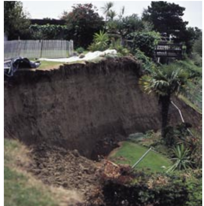
A steep backyard fill slope has failed, creating great financial hardship for the affected homeowner.
