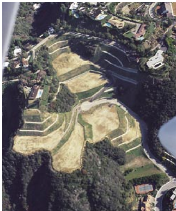
Concrete bench and down drain systems need to be maintained year-round.
