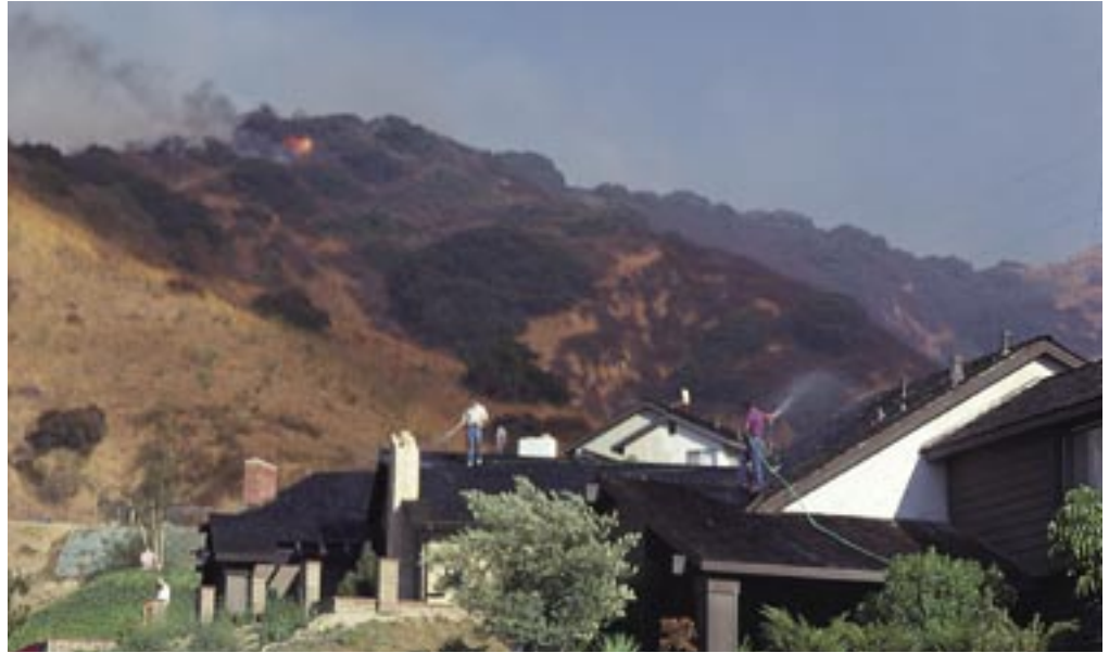
Wood shingle roofs require an inappropriate amount of manpower and water during a wildfire because they are easily ignited by flying sparks.
