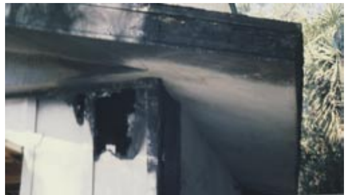
Boxed eaves that prevent heat entrapment even if the wood siding catches on fire.
