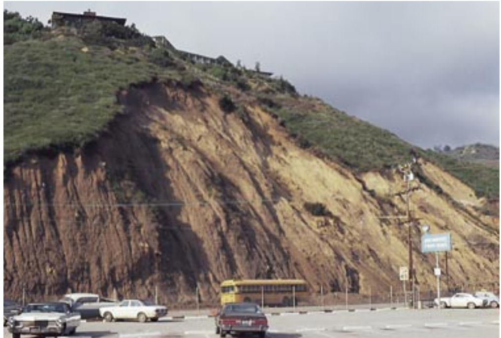
Steep slopes undercut by roads are especially susceptible to slips and slides.
