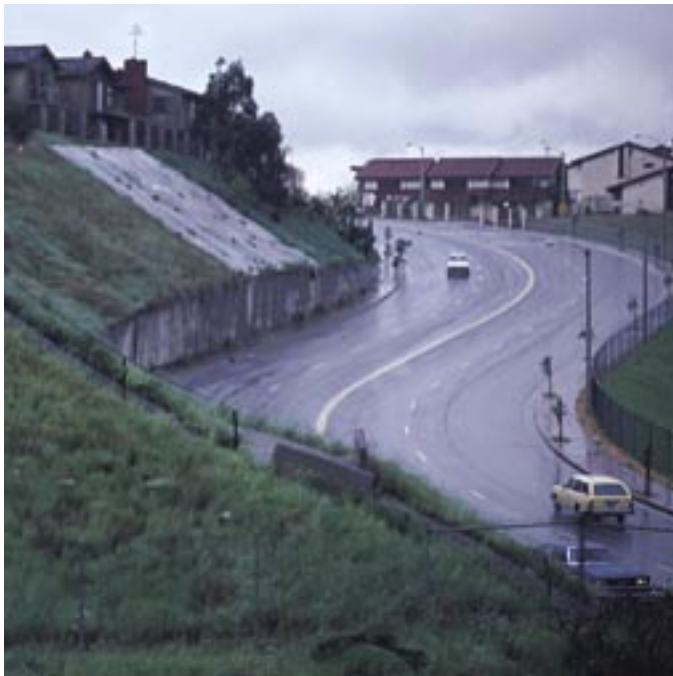
The plastic is well anchored and covers the whole slope.
