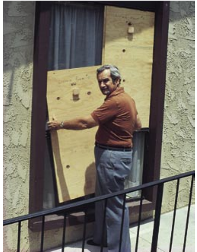
Shutters, even emergency plywood shutters, that protect windows.
