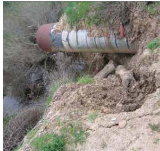
Photo 43: Improperly installed culverts can create areas of severe erosion
