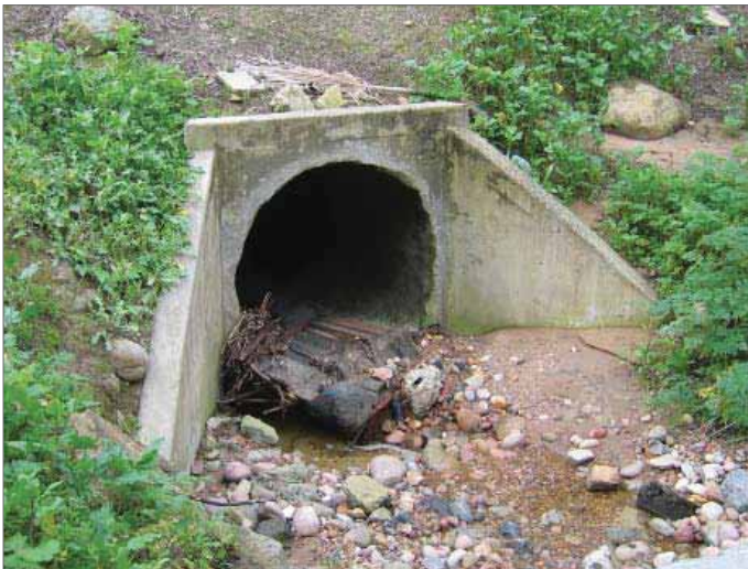
Photo 42: Debris can cause blockages
