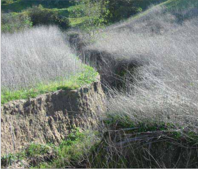
Photo 40: Large gullies have formed below many storm drain outfalls
