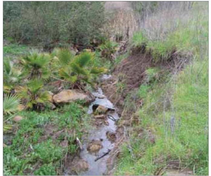
Photo 41: Streambank erosion is common downstream of storm drain outfalls
