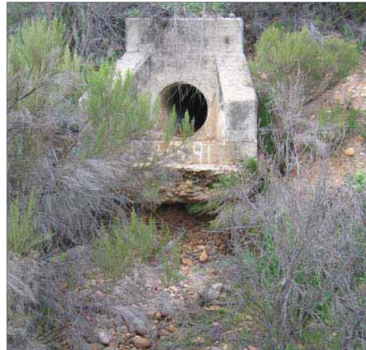
Photo 39: Storm drain outfall showing severe erosion downstream due to high water velocities
