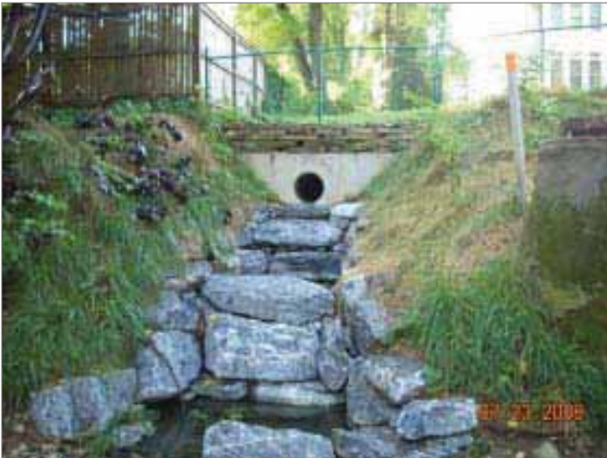
Photo 38: Sample Storm Drain BMP to slow water velocities and reduce erosion
