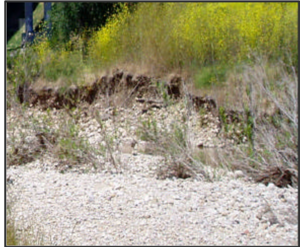
Figure 8. Stream bank erosion
