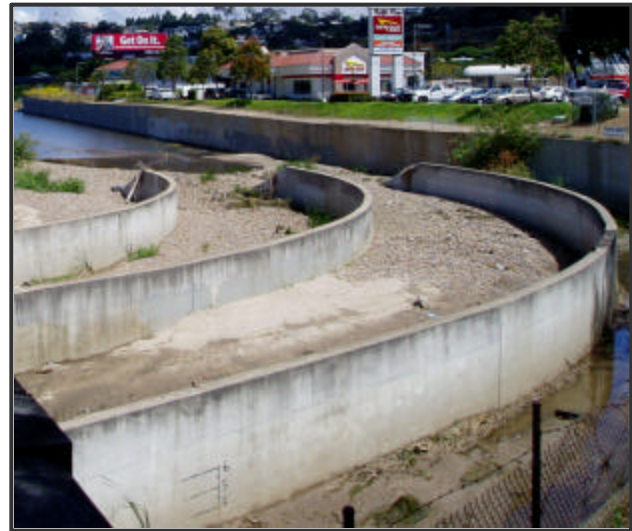
Figure 4. Vertical walled concrete channel of Rose Creek at East Mission Bay Drive
