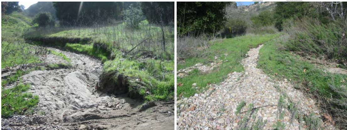
Figure 2-5. Utility erosion
