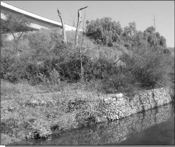
Figure 52: Gabion streambank protection in San Clemente Canyon near Genesee on-ramp
