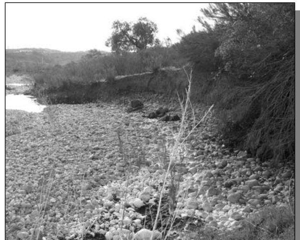
Figure 33: Active bank erosion on outer bend upstream of Interstate 805 in Rose Canyon
