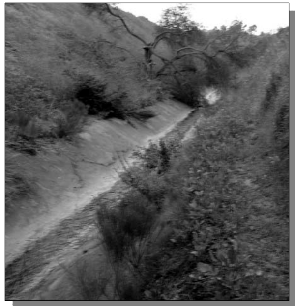
Figure 57: Concrete V-ditch channel in Lakehurst Canyon
