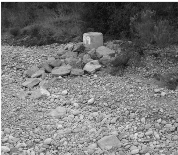
Figure 42: Streambed erosion threatened sewer manhole that is now protected with riprap in Rose Canyon
