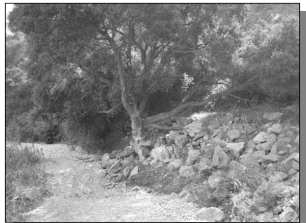
Figure 51: Streambank armoring with riprap upstream of old railroad bridge in Rose Canyon
