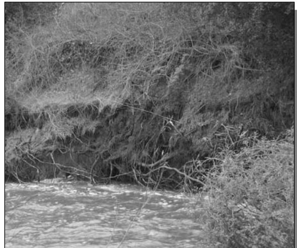
Figure 37: Active bank erosion during storm flows below confluence
