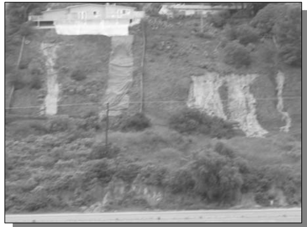
Figure 64: Slope failures related to iceplant and storm runoff from residences in Gilman Canyon
