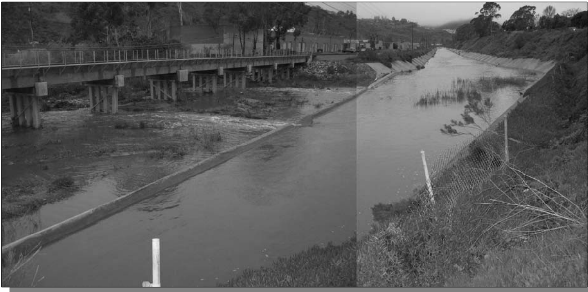
Figure 60: Concrete trapezoidal channel above Santa Fe Street crossing looking upstream
