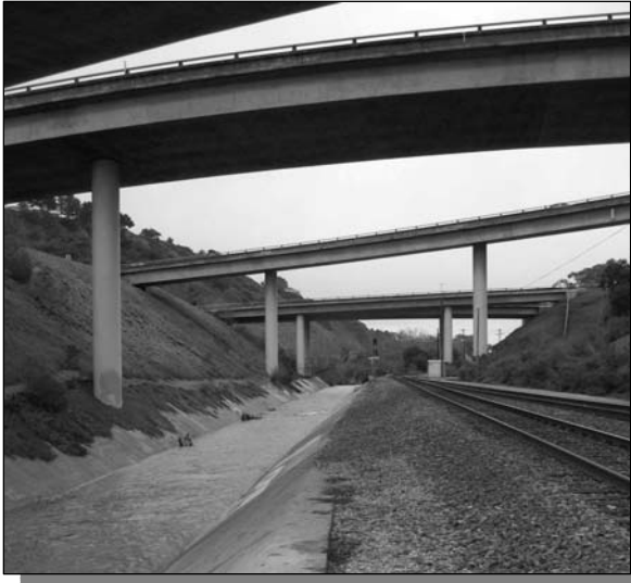
Figure 58: Concrete trapezoidal channel running underneath interchange between Interstate 5 and State Route 52
