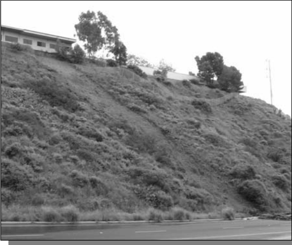
Figure 63: Slope failure related to iceplant and storm runoff below residential development
