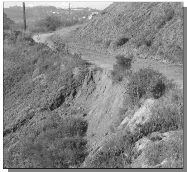
Figure 62: Slope failure related to iceplant along railroad access road in Rose Canyon
