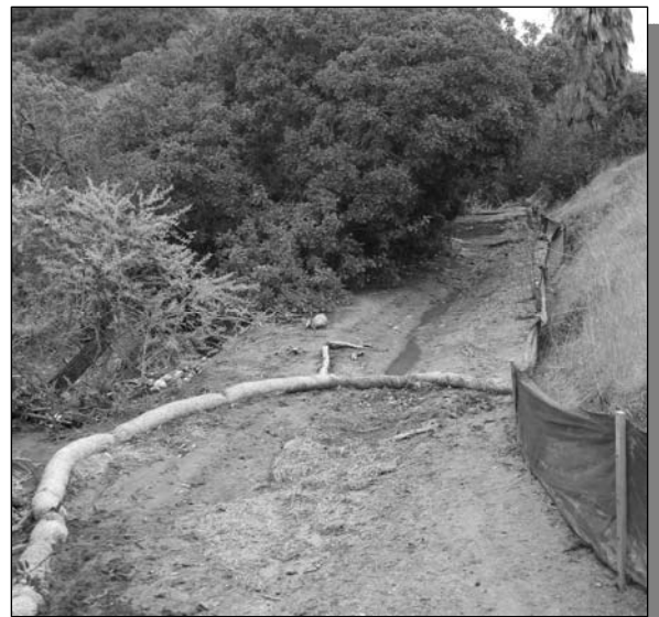
Figure 31: Sewer access road erosion and corrective best management practices below storm drain outfall
