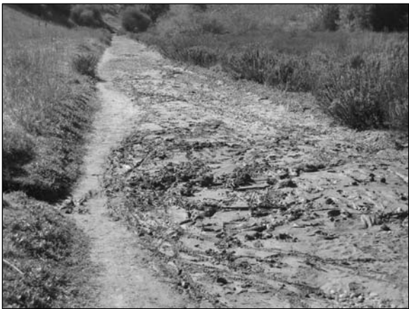
Figure 44: Sediment flowing onto Rose Canyon trail/access road from eroding storm drain channel
