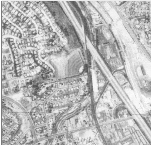
Figure 14: Recently constructed USACE concrete box channel
