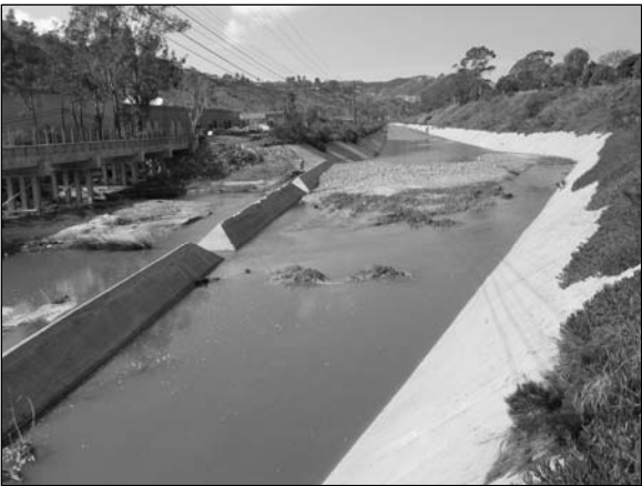
Figure 48: Depositional bar formed on inside of channel bend behind concrete flow diverter in lower Rose Creek
