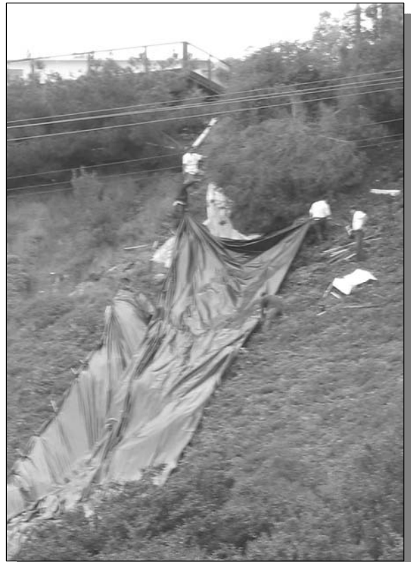
Figure 66: Slope failure related to iceplant and storm runoff from residence in Gilman Canyon
