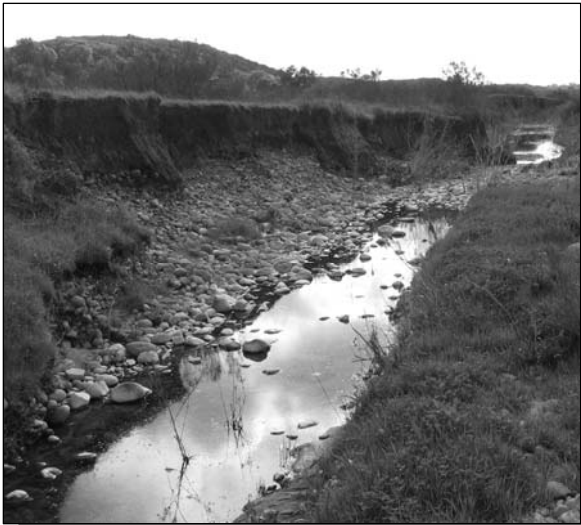
Figure 32: Active bank erosion upstream of Interstate 805 in Rose Canyon
