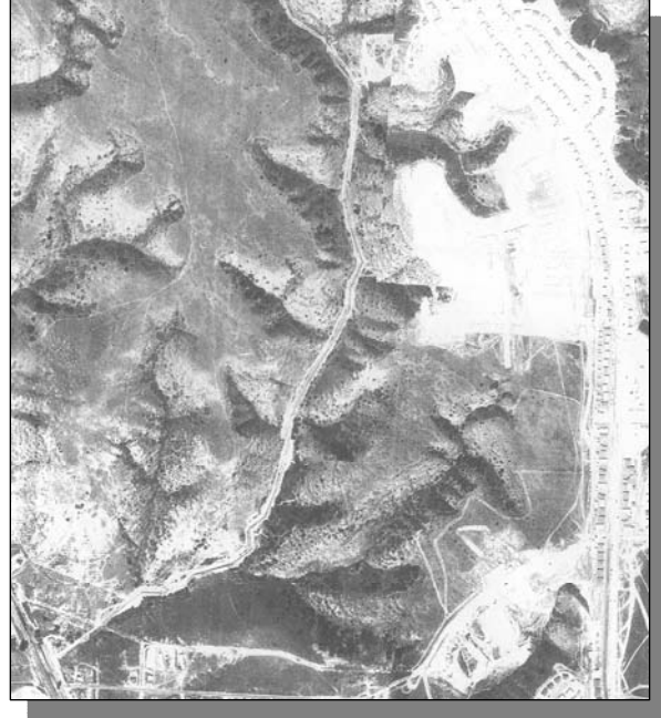
Figure 9: Sewer main being constructed in Stevenson Canyon
