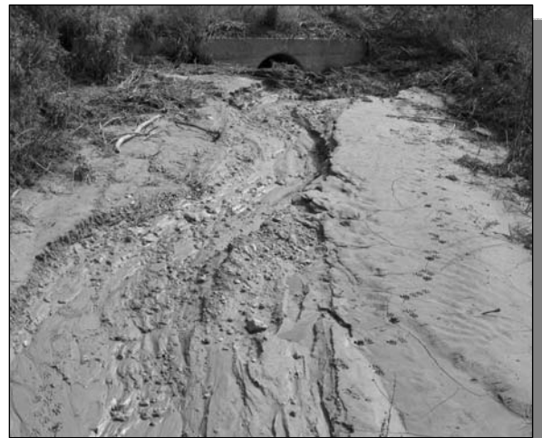
Figure 45: Sediment deposition on upstream side of culvert in Rose Canyon just north of State Route 52
