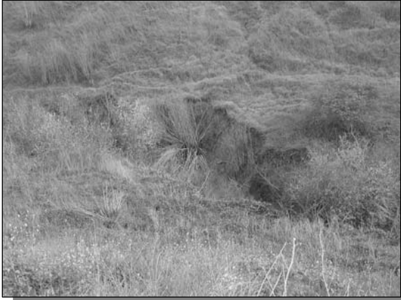
Figure 40: Tributary drainage along Rose Canyon that has experienced significant down-cutting (10-15ft) over the past 40 years
