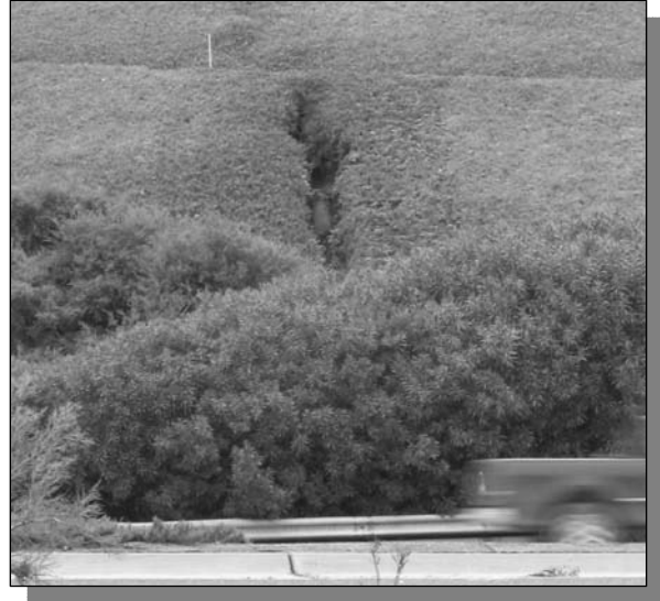
Figure 29: Storm drain related gully erosion along Interstate 5
