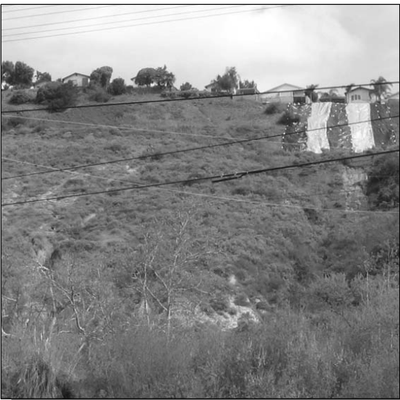
Figure 65: Slope failures related to iceplant and storm runoff from residences in Rose Canyon
