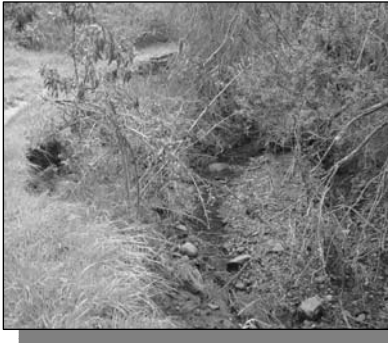
Figure 1: Eroding streambank and bed in Lakehurst channel
