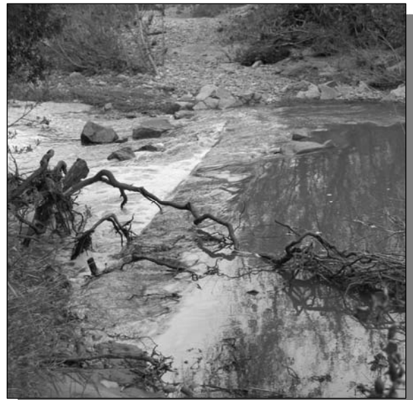
Figure 43: Concrete protect sewer main crossing Rose Creek below confluence being exposed by streambed erosion
