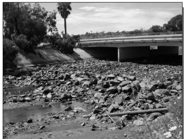
Figure 55: Concrete streambank protection and riprap streambed at Grand Ave crossing
