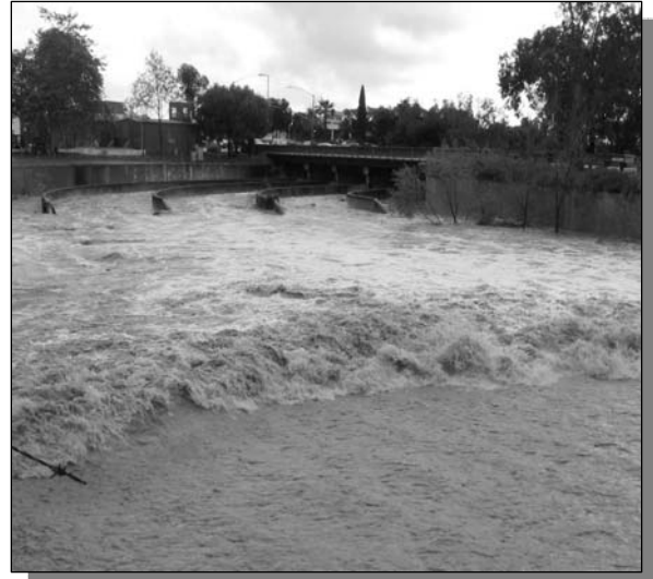
Figure 59: Concrete box channel between Interstate 5 and Mission Bay Drive during a storm event
