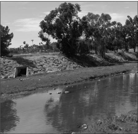
Figure 54: Riprap streambank protection along lower Rose Creek
