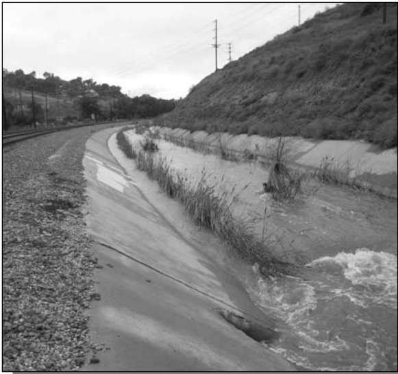
Figure 56: Upstream most concrete trapezoidal channel along railroad tracks north of State Route 52
