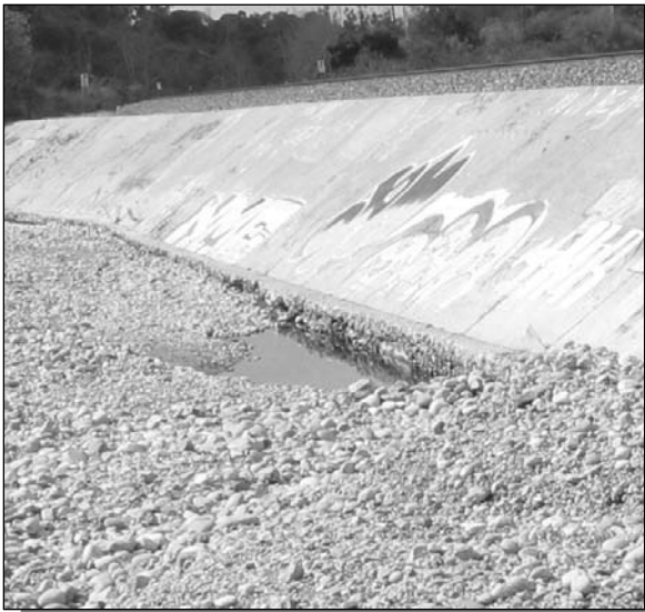
Figure 38: Streambed erosion undercutting concrete bank protection along railroad tracks in Rose Canyon
