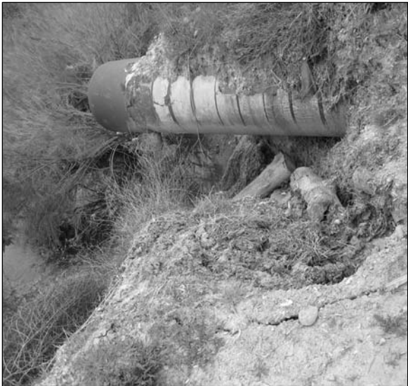
Figure 26: Eroded culvert in Rose Canyon
