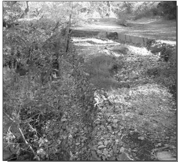
Figure 53: Gabion streambank protection to protect sewer main in San Clemente Canyon
