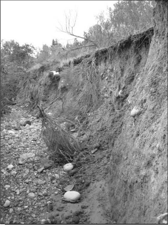
Figure 34: Active bank erosion in Stevenson Canyon
