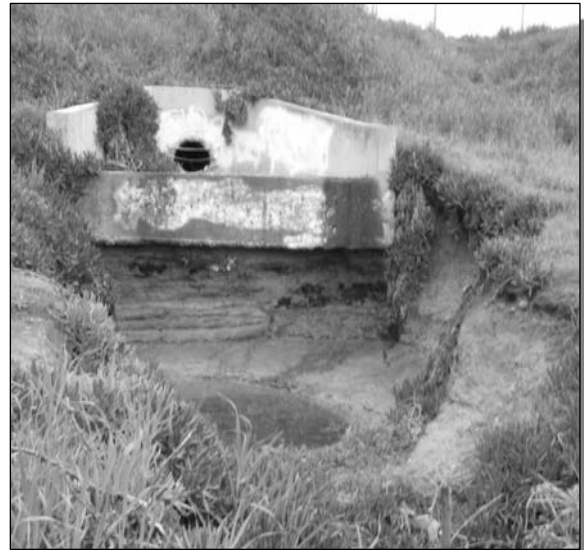
Figure 27: Eroded outfall in tributary canyon below elementary school
