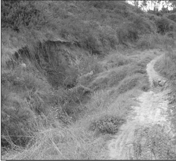
Figure 28: Erosion downstream of storm drain outfall in tributary to Rose Canyon
