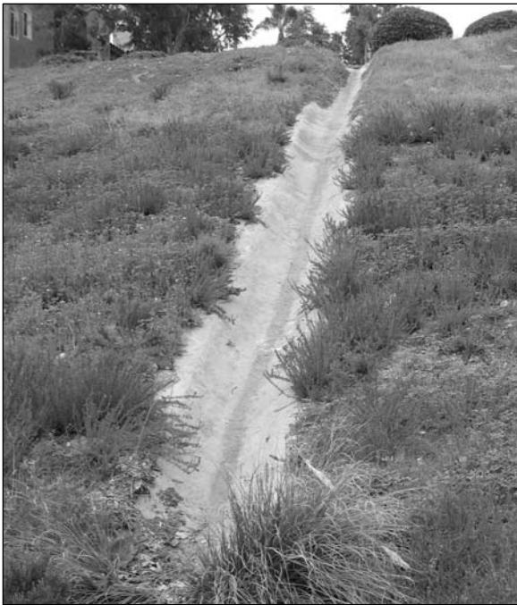
Figure 30: Concrete V-ditch draining condominium complex
